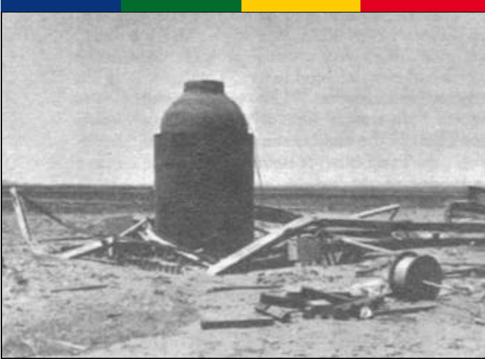
Jumbo stands unscathed, its tower crumpled around it.
