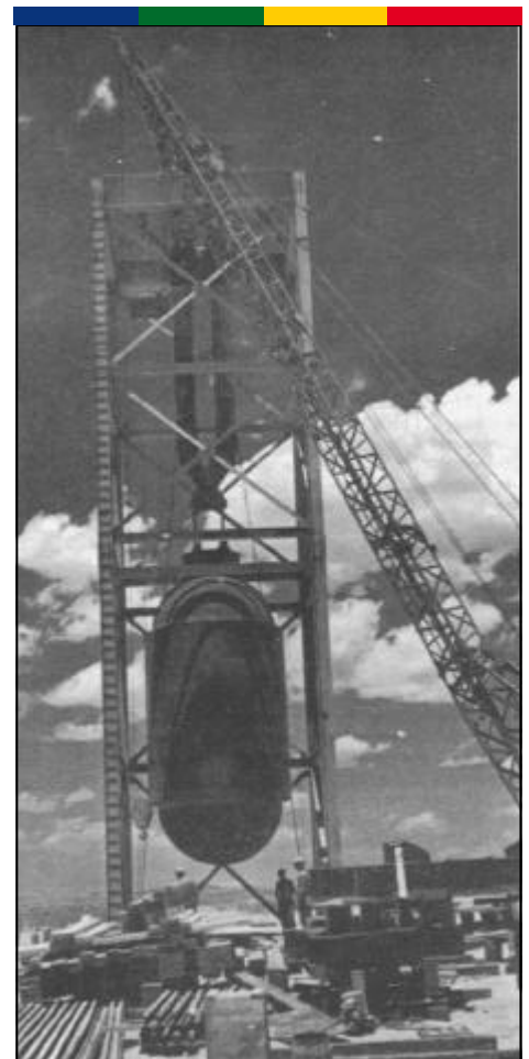
At Trinity, Jumbo was erected on a tower 800 feet from Ground Zero. It survived the explosion unscathed.
