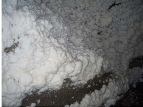
Figure 5: Salt deposits on the walls of the tunnels of Wieliczka Salt Mine.
